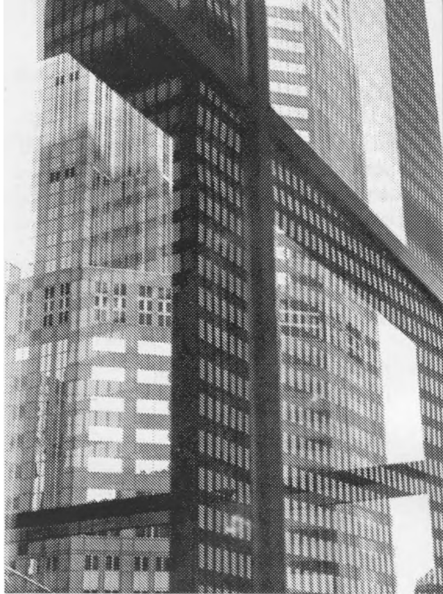
Sears Tower and 311 South Wacker Drive Building, Chicago, Illinois.
