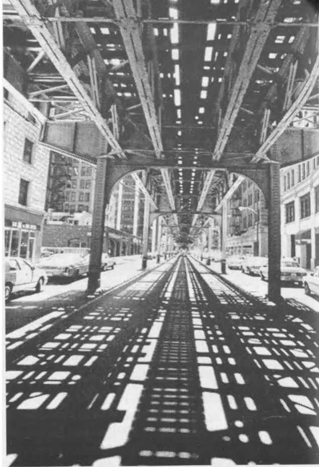
The elevated track on Wells Street, Chicago, Illinois
